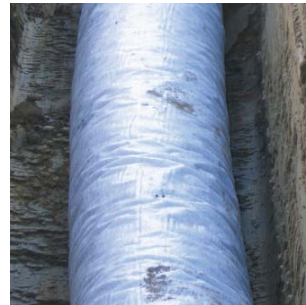
Polybed system wrapped in non-woven needle punched geotextile, which is factory fitted
