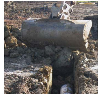
Arisings used to backfill to top of trench
