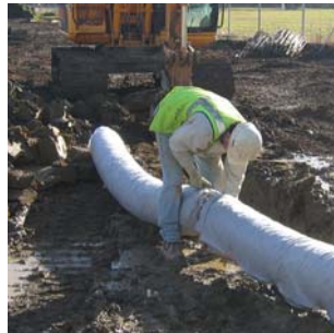
Polybed system installed into dug trench
