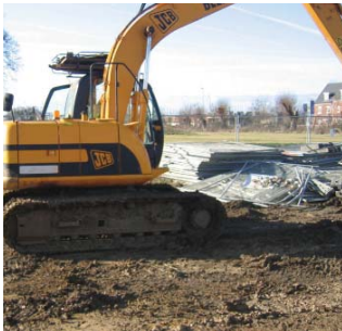
Trench excavated to site specific requirements arisings kept for re-use
